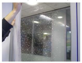
If necessary fix the bubble wrap in place with tape.
