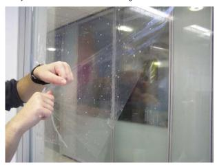
For a double layer construction of 8150 it is best to first warm up the film with an infrared lamp to about 30 - 40°C. Make sure with the infrared thermometer that the temperature of the glass is not higher than 50°C. Be careful if the temperature variation of the glass changes too much in a short time it could get damage.
